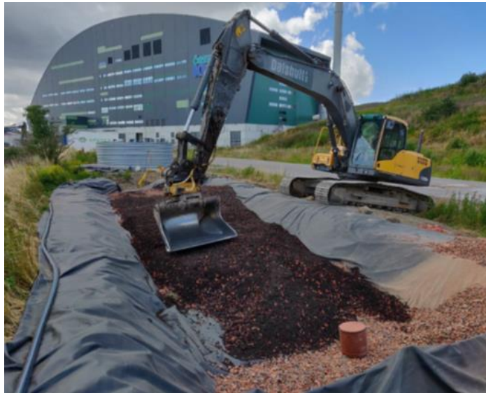
Figure 10 Contrtruction of the hybride filter
