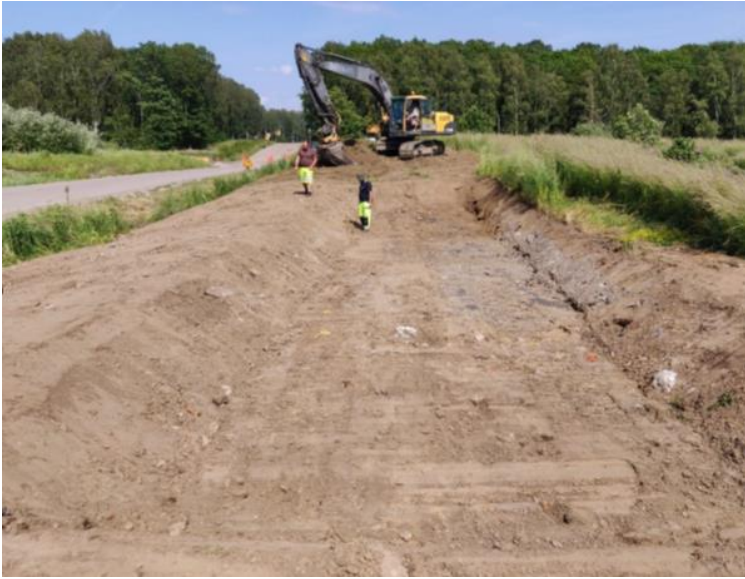
Figure 7 Construction of hybride filter (ground work)
