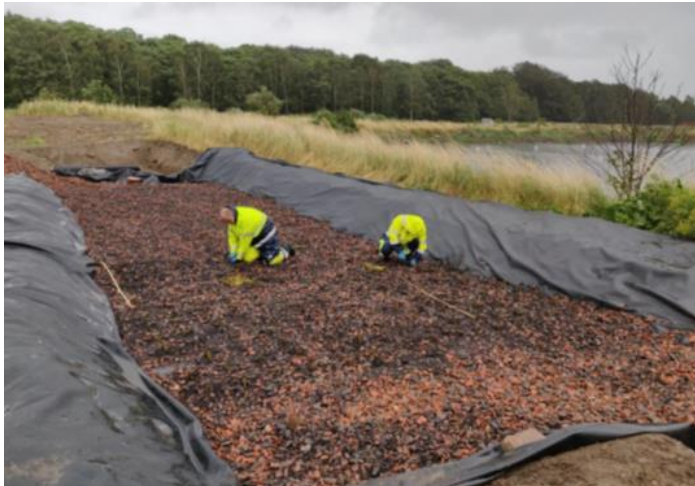
Figure 11 Construction of hybrid filter, planting of Salix
