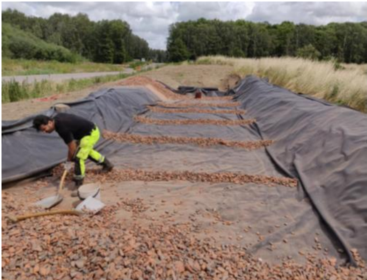
Figure 8 Construction of hybride filter (brick material)
