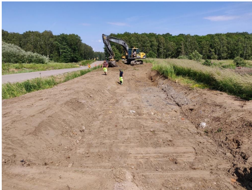
Figure 9 Construction of Laqua 2 system
