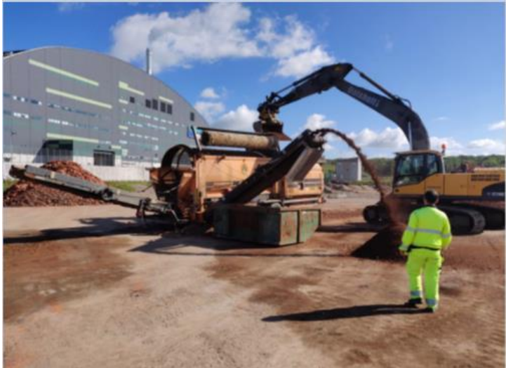
Figure 8 Construction of hybride filter (brick material)
